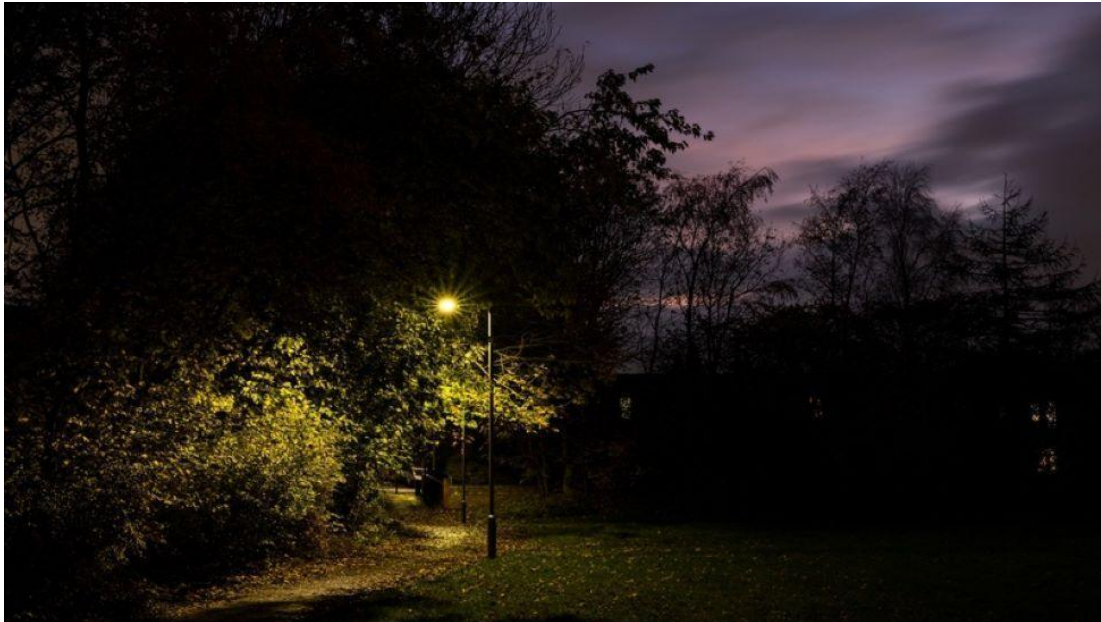
Figure 26 – Baronscourt Park, Edinburgh hybrid street lighting.
